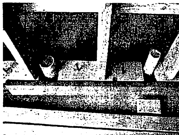
Plumbing penetrations through plates
