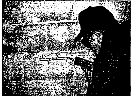
Apply thick bead to walls
